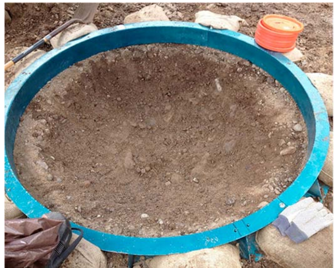
FIG. 4 Test Pit Excavation
